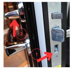
The door locks when the door knob is in right position and the button is up. The door doesn't close with a key. Remember to take the key with you when going outside!
